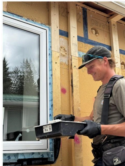
Figure 13. Holes are drilled through the rigid wood fibre panel into each cavity and into the space above each panel. Hoses are inserted in 3 or 4 cavities ahead of the one being filled. As each cavity is filled the hose is leap frogged ahead and the panel is filled with dense packed wood fibre. Afterwards a glue and a tape are applied to seal up the holes.
