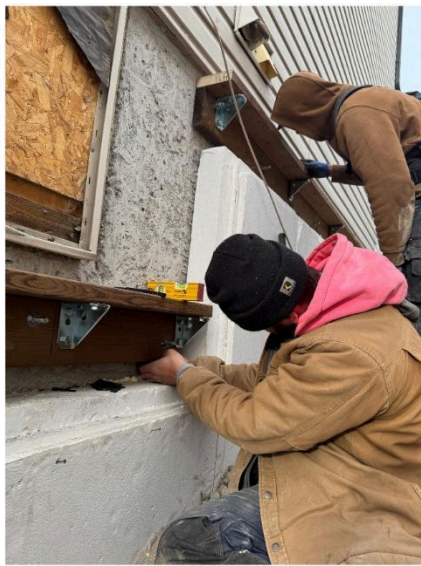
Figure 17. The new ledger design (left) featuring treated wood and over the counter hardware is better than the steel one (right) used on this project. It was cheaper, easier, and has lower embodied carbon.
