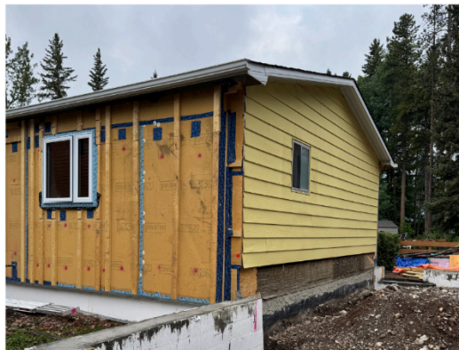
Figure 10. The PEER panel installation is completed except for siding, the foundation for the ADU is poured, the untouched wall was addressed when the ADU was completed.
