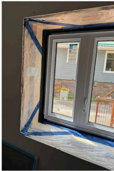
Figure 7. The interior of the window is connected to the existing polyethylene air/vapour barrier with high quality tapes. The exterior of the window is connected to the weather resistive barrier with high quality tapes.
