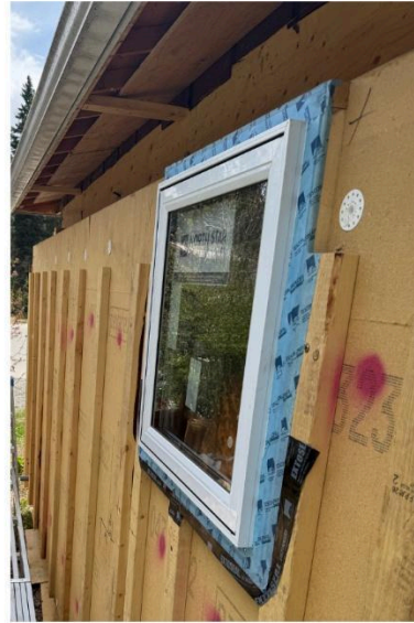
Figure 7. The interior of the window is connected to the existing polyethylene air/vapour barrier with high quality tapes. The exterior of the window is connected to the weather resistive barrier with high quality tapes.
