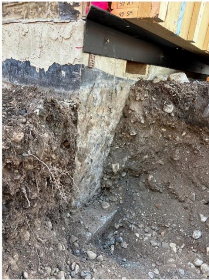
Figure 12. The steel ledger was fixed to the concrete foundation; the ledger was screwed to the PEER panel through pre-drilled holes. The top of the panel was fixed to the existing structure using angle brackets. Plywood and framing were attached to the roof truss.
