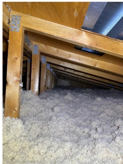
Figure 9. Leaks in the air/vapour barrier were repaired and wood fibre was blown into the attic making sure to maintain ventilation.
