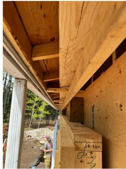
Figure 12. The steel ledger was fixed to the concrete foundation; the ledger was screwed to the PEER panel through pre-drilled holes. The top of the panel was fixed to the existing structure using angle brackets. Plywood and framing were attached to the roof truss.
