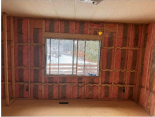
Figure 2. 2" by 4" stud wall construction with 1" by 4" notched in above polyurethane vapour barrier. Aluminium windows had poor energy performance and leaked air.
