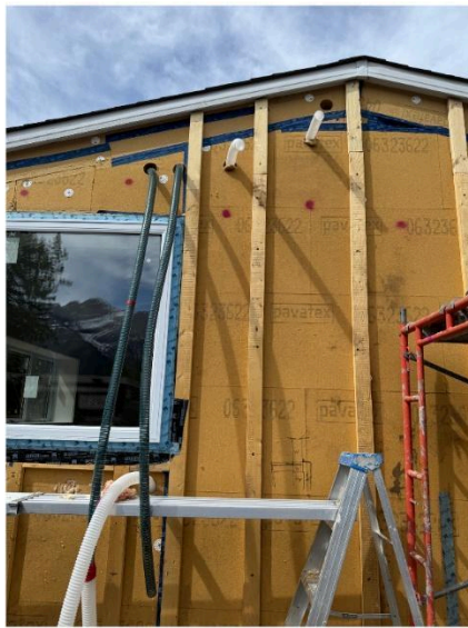
Figure 13. Holes are drilled through the rigid wood fibre panel into each cavity and into the space above each panel. Hoses are inserted in 3 or 4 cavities ahead of the one being filled. As each cavity is filled the hose is leap frogged ahead and the panel is filled with dense packed wood fibre. Afterwards a glue and a tape are applied to seal up the holes.
