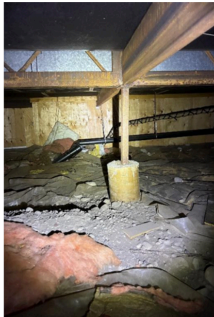
Figure 1. Vented crawlspace features a dirt floor, concrete walls covered with Styrofoam and plywood, steel structural elements, heating system ductwork, and the sewer drain system.
