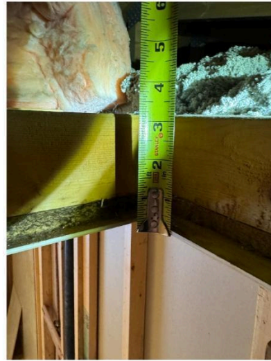
Figure 3. Standard attic build up with minimal insulation. Leaks were repaired and blow-in wood fibre to be added.
