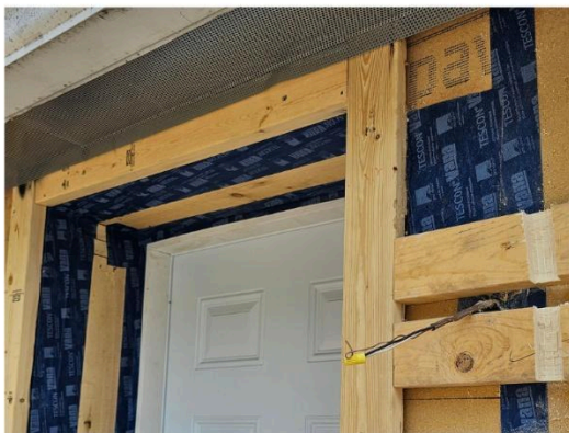
Figure 8. Doors are connected to the Air/vapor barrier on the inside and the weather resistive barrier on the outside using high quality tapes.
