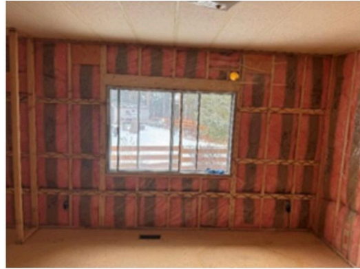
Figure 2. 2" by 4" stud wall construction with 1" by 4" notched in above polyurethane vapour barrier. Aluminium windows had poor energy performance and leaked air.
