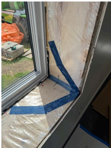
Figure 16. Two different strategies for window interiors. One featured plywood, while the other featured metal mending plates. The mending plates were quicker and just as effective.
